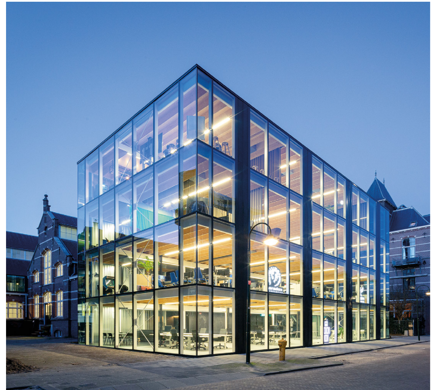
Photo: Bouwdeel D, a fully demountable office building in Delft, constructed entirely from a prefabricated steel structure and prefabricated laminated wooden floors of Laminated Veneer Lumber (LVL) elements. Credits: cepezed
